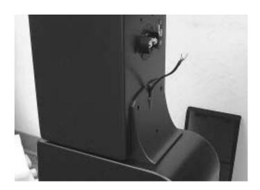
Step 8: Connecting the Monitor Connection Harness to the Monitor
